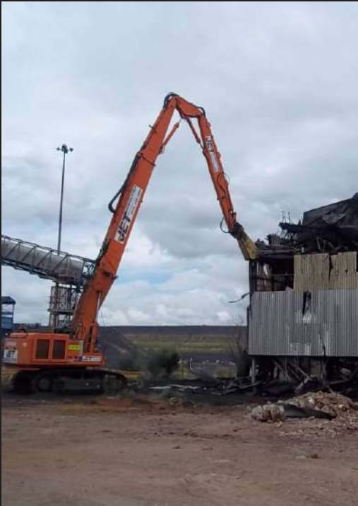
▲▲▲▲▲▲▲▲▲▲▲▲▲▲▲▲ Mechanical Demolition of PSS Plant
