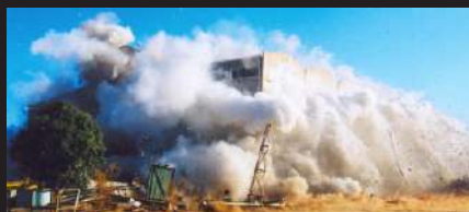
Explosive Demolition of Large Concrete Mill Building
