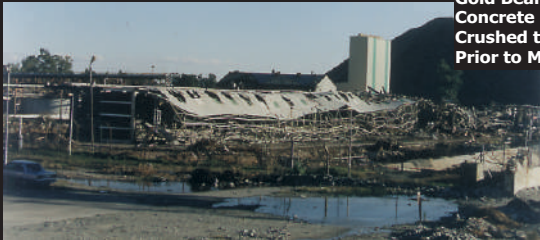
Explosive Demolition of an Unusually Long Steel Structure (7 storeys high x 250 m long)
