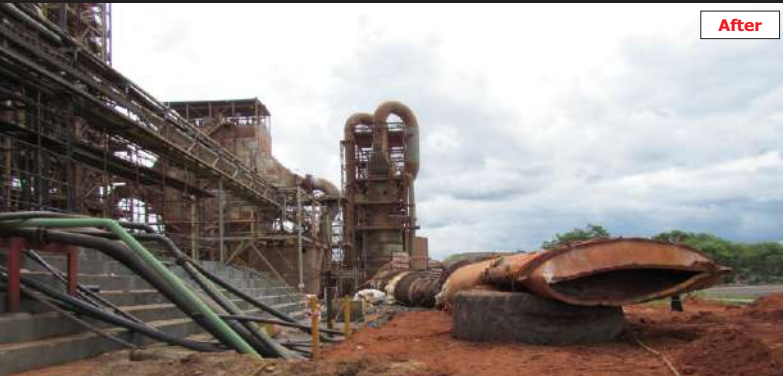
Partial Demolition of Operating Gold and Acid Plant Including Controlled Topping of 71 m High Stack Within 2 m of an Active Plant and Equipment
