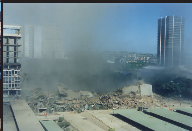
Implosion of the Fire Damaged Munitoria Building in Pretoria City Centre Using 300 kg of Explosives. Removal of 44 000 Tonnes of Rubble Was Done in 25 days. The Entire Project Was Completed in 3 Months
