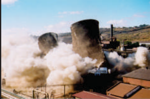
Sequential Explosive Demolition of 5 Concrete Cooling Towers
