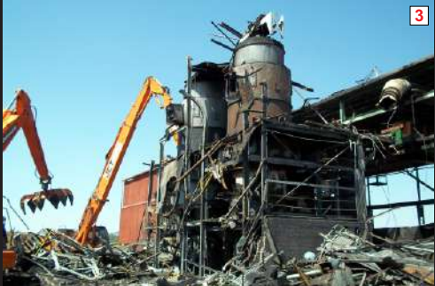
Demolition of 3 Gas Producers Located 1 m from a Storage Building Which Remained
