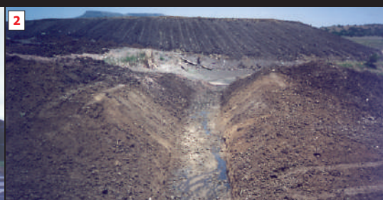
▲▲▲▲▲ Turnkey Project : (1) Plant Demolition; (2) Reshaping and Soil Cladding of Waste Dump Involving 300 000 m 3 of Earthmoving; Installation of Surface Diversion Canals, Subsurface Drains and Evaporation Ponds; (3) Rehabilitation and Establishment of Grass
