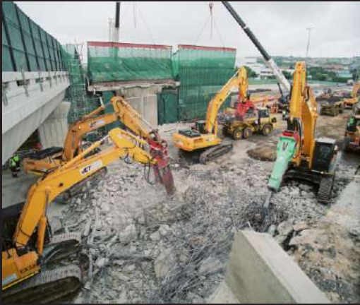
Overnight Demolition and Removal of 3 Large Bridges on the N1 Motorway Between Johannesburg and Pretoria
