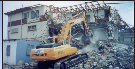
Mechanical Demolition of Commercial Buildings
