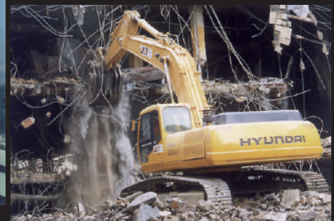
Clean Up of the Fire Damaged Munitoria Building Prior to Blasting. A Total of 1 500 Tonnes of Burnt Debris Was Removed
