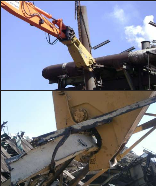
▲▲▲▲▲▲▲▲▲▲▲▲▲▲▲▲ Cold Cutting of Industrial Plants Using Specialised Hydraulic Shears
