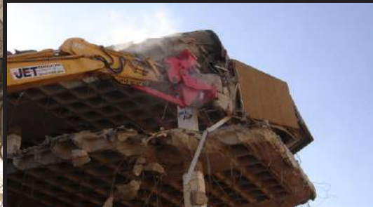
Mechanical Demolition of Commercial Buildings
