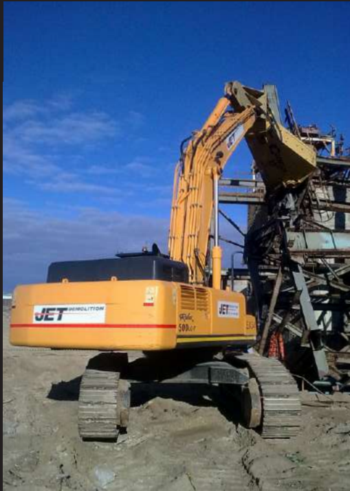
▲▲▲▲▲▲▲▲▲▲▲▲▲▲▲▲ Demolition of Heavy Steel Crusher Structure by a Large Hydraulic Shear
