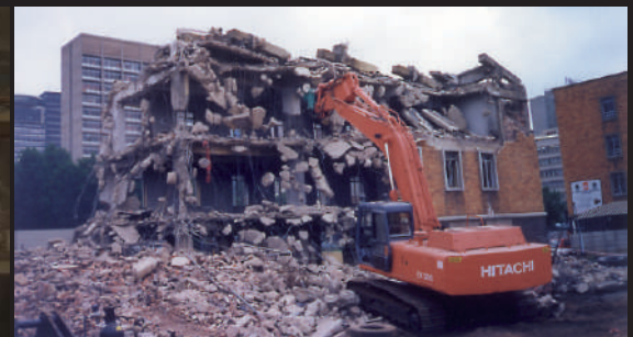
Mechanical Demolition of Commercial Buildings
