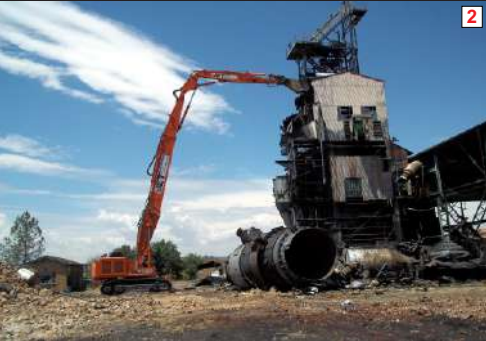
Safe Top-Down Demolition of Chimney
