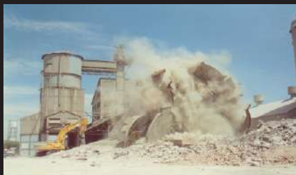
Controlled Mechanical Dropping of Clustered Cement Silos
