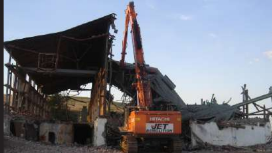
High Reach Excavator Demolishing Mine Shaft Winder House
