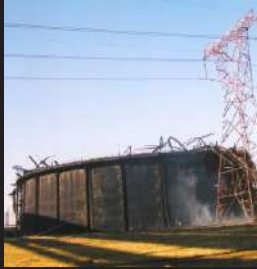
Explosive Demolition of a 68 m High Fire Damaged Gas Holder Adjacent to Main Plant Power Line and Gas Line
