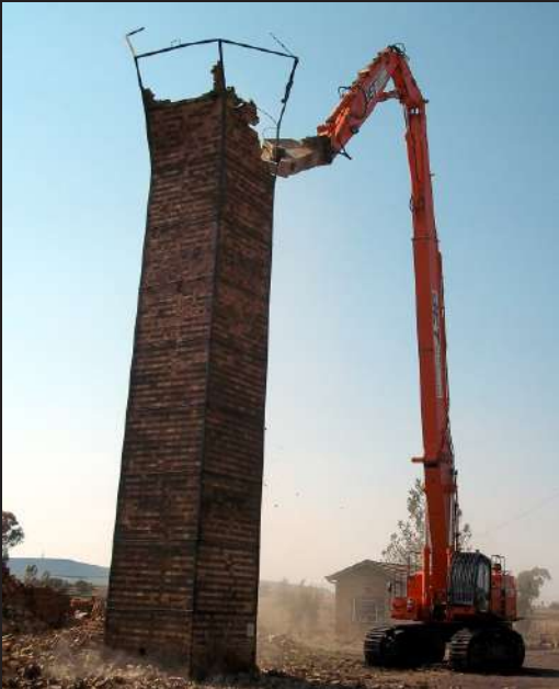
Safe Top-Down Demolition of Chimney
