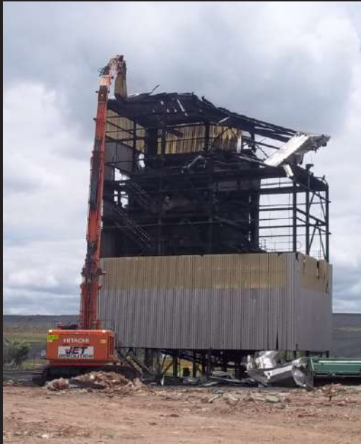
Mechanical Demolition of Plant Using Specialised High Reach Machine
