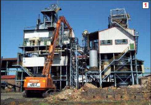
Controlled Demolition of Building Containing Fully Operational Municipal Substation
