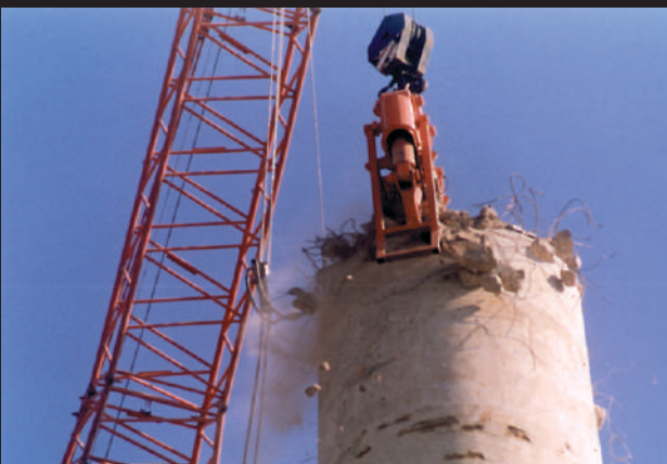
Innovative Demolition of a 76 m High Concrete Chimney in Only 7 Days at an Oil Refinery Using a 1 000 Tonne Crusher Suspended from a 440 Tonne Crane. Blasting Was Not an Option Because of Insufficient Space and Safety Considerations
