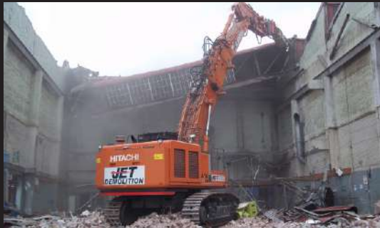
Controlled Demolition of Steel & Concrete Structure Adjacent to Operating Gas Plant
