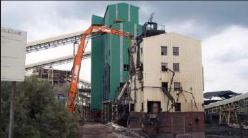
Demolition of 3 Gas Producers Located 1 m from a Storage Building Which Remained
