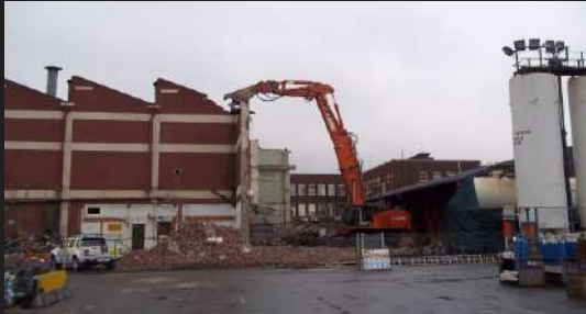
Mechanical Demolition of Plant Using Specialised High Reach Machine
