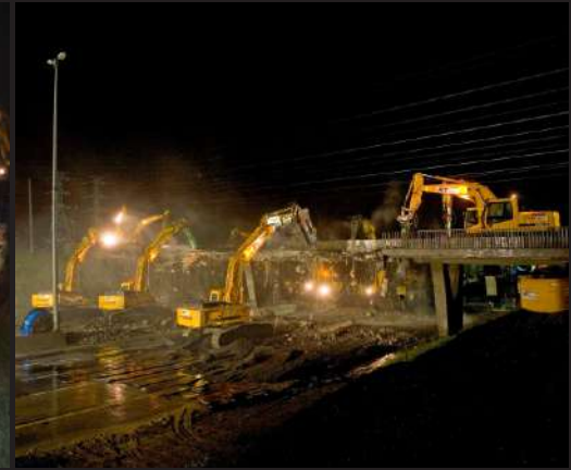
Overnight Demolition and Removal of 3 Large Bridges on the N1 Motorway Between Johannesburg and Pretoria
