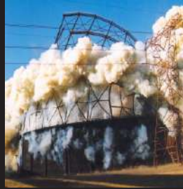
Explosive Demolition of a 68 m High Fire Damaged Gas Holder Adjacent to Main Plant Power Line and Gas Line
