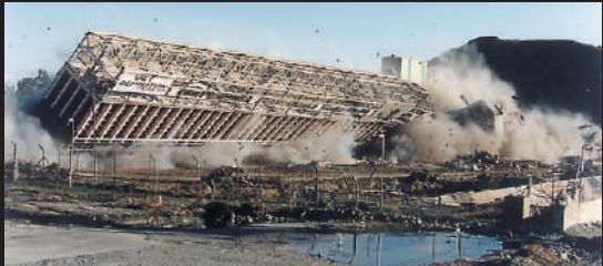
Explosive Demolition of an Unusually Long Steel Structure (7 storeys high x 250 m long)
