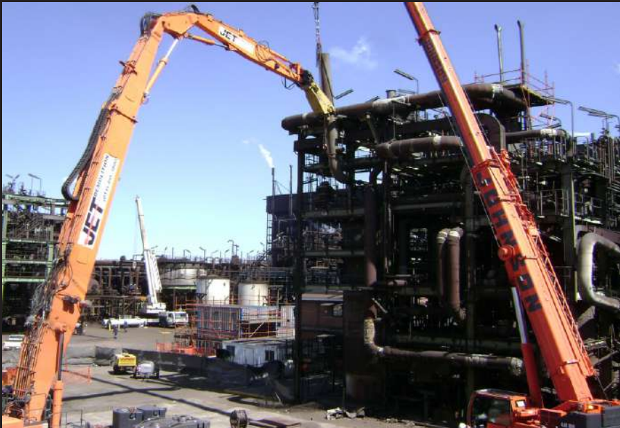
▲▲▲▲▲▲▲▲▲▲▲▲▲▲▲▲ Cold Cutting and Rigging of Petrochemical Plant in Active Process Area that Prohibits Hotwork
