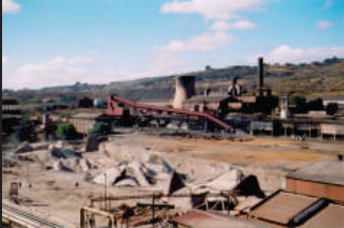
Sequential Explosive Demolition of 5 Concrete Cooling Towers
