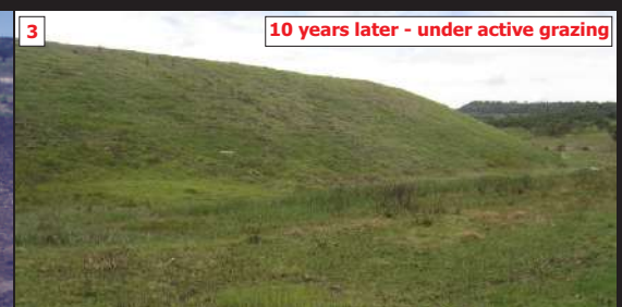
▲▲▲▲▲ Turnkey Project : (1) Plant Demolition; (2) Reshaping and Soil Cladding of Waste Dump Involving 300 000 m 3 of Earthmoving; Installation of Surface Diversion Canals, Subsurface Drains and Evaporation Ponds; (3) Rehabilitation and Establishment of Grass
